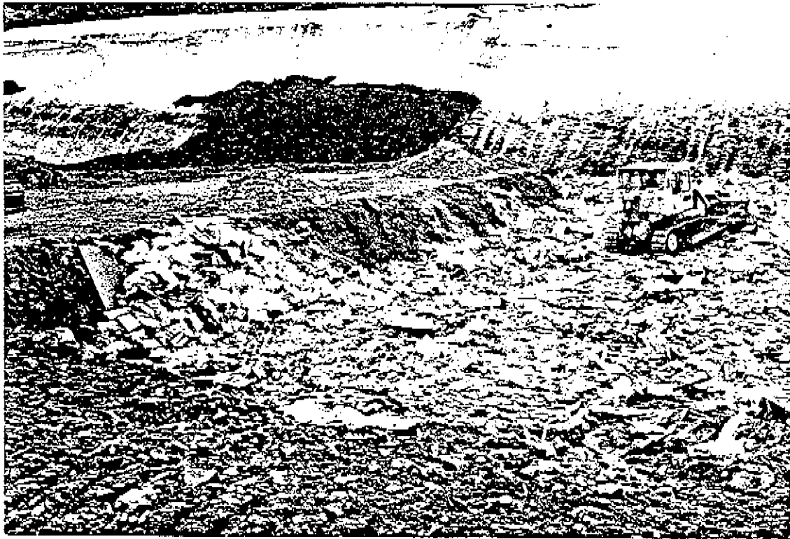
figure 7 Tractor compaction at a modified landfill
