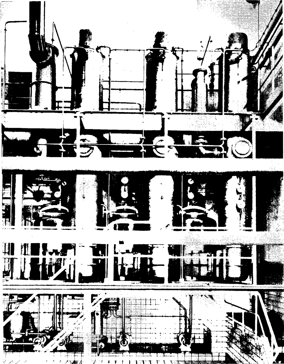
FIG. 3 FALLING-FILM EVAPORATOR, THREE EFFECTS
